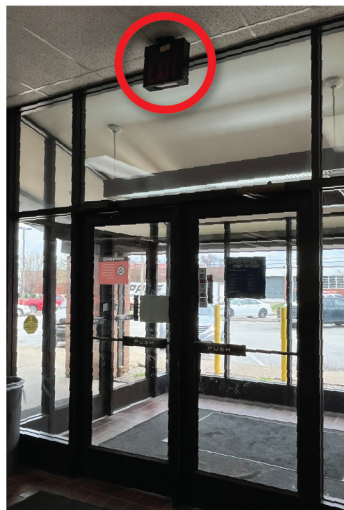
Emergency Exit Light Not Illuminated
