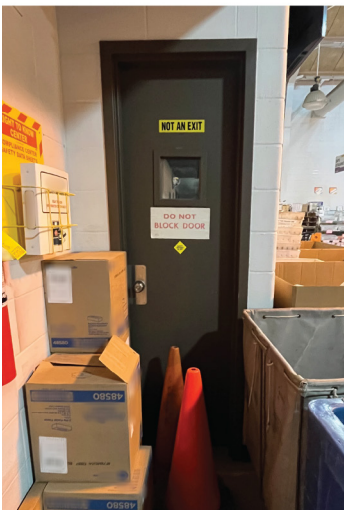
Blocked Inspection Service Door
