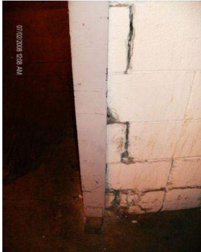
Illustration 6: On July 2, 2008, at 12:08 a.m., we observed damage to a wall in the Providence P&DC caused by a vehicle impact.
