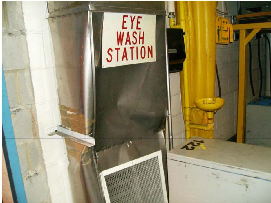
Illustration 2: On April 28, 2008, at 2:08 p.m., we observed damage to a duct and wall in the Raleigh P&DC, caused by a vehicle impact.
