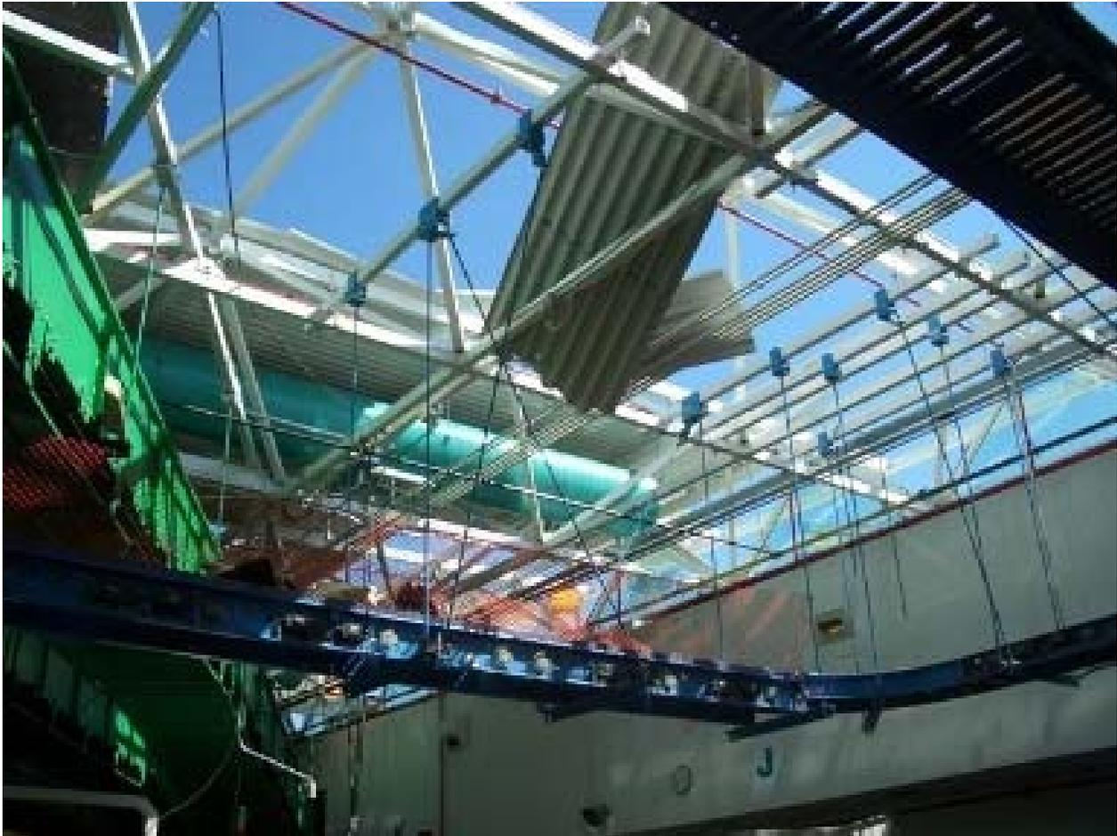
**Miami AMC Roof with Sections Missing**
